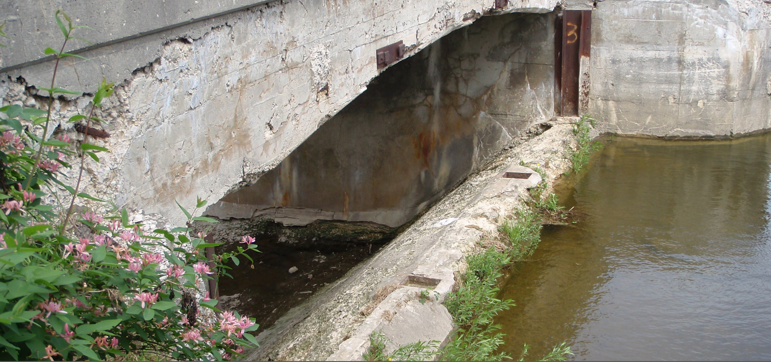
Howson Dam – North Maitland River
